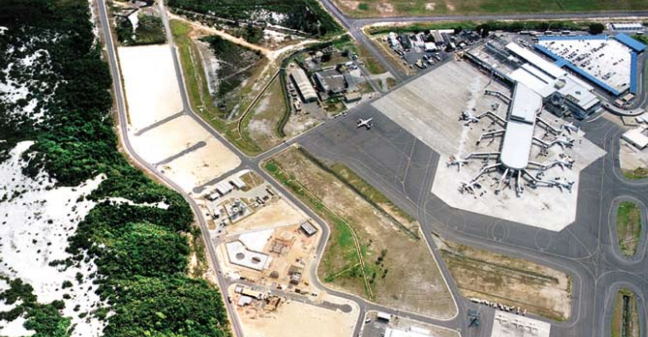
Aeroporto Internacional de Salvador Salvador International Airport
